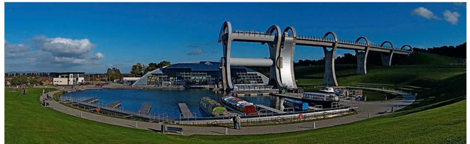
Figure 19. The Falkirk Wheel a rotating boat lift in Scotland, connects the Forth and Clyde Canal with the Union Canal. The lift, named after the nearby town of Falkirk, opened in 2002.
